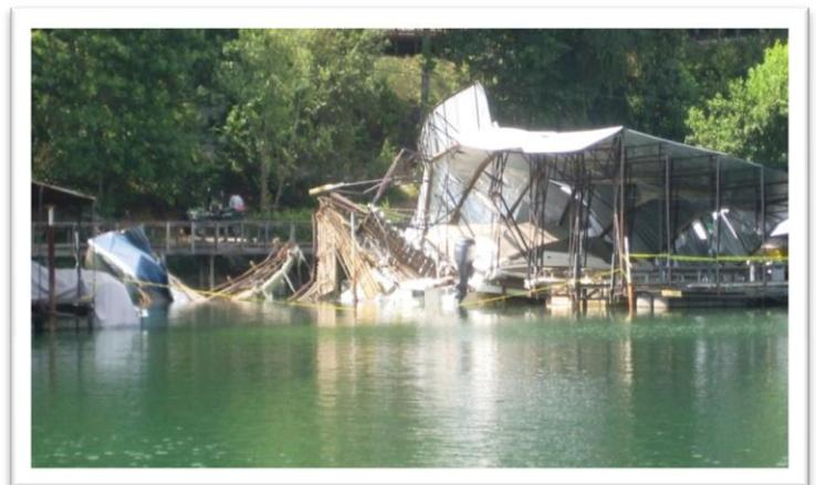
We occasionally hear severe thunderstorm warnings and sometimes they mention high winds. A microburst (small, focused downburst from a severe thunderstorm) probably caused this dock damage at Mountain Harbour Marina. It is amazing how powerful the wind must have been and how limited was the area of damage.
